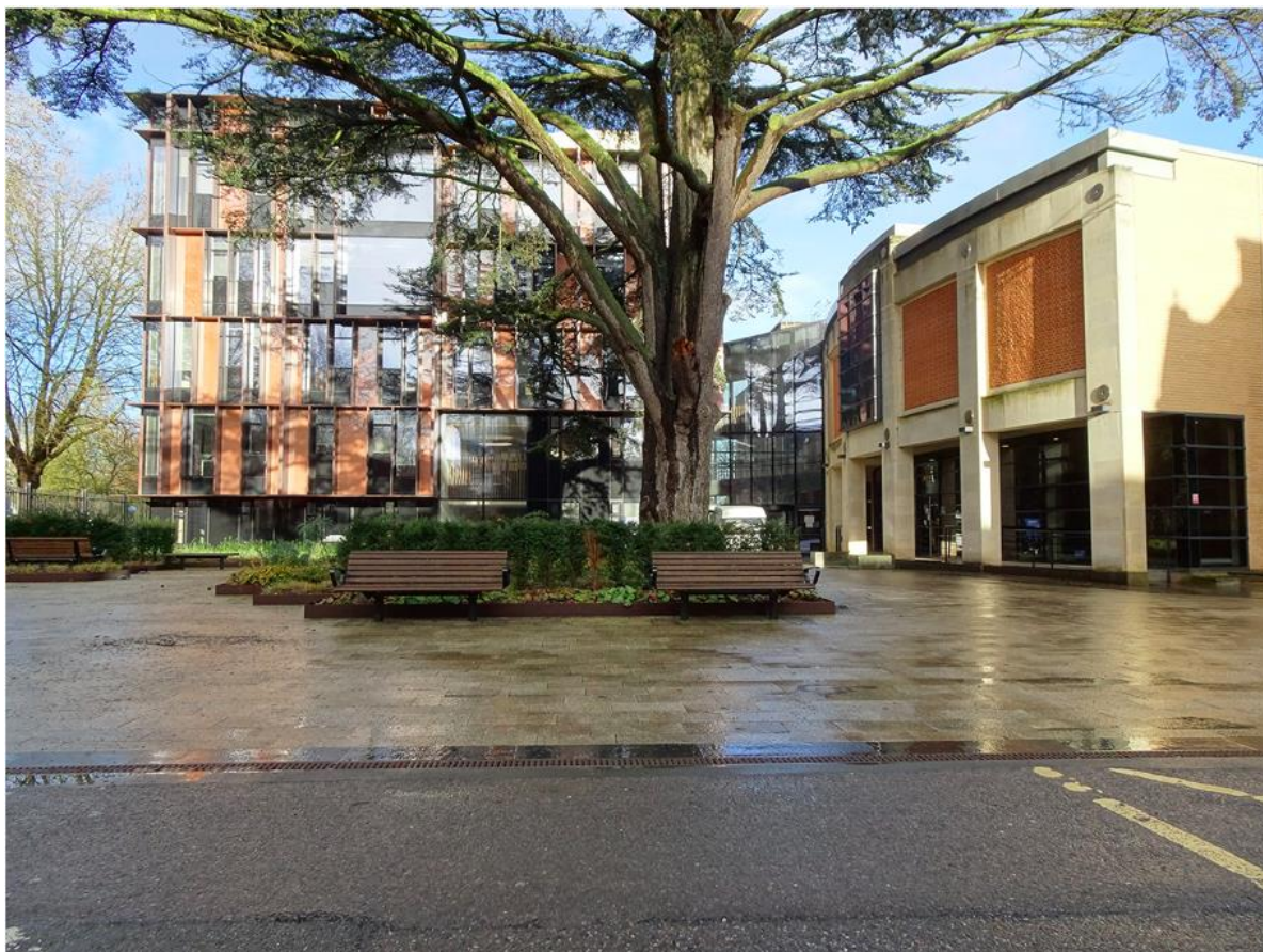
An external view of the Clarendon Quad, with the Beecroft Building (centre) and Martin Wood Lecture Theatre (right)
